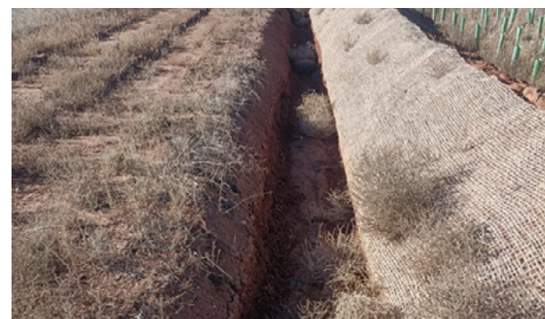
Implementation of coconut mesh to prevent PV erosion "Valdenebro Solar" Muniesa (Teruel)
